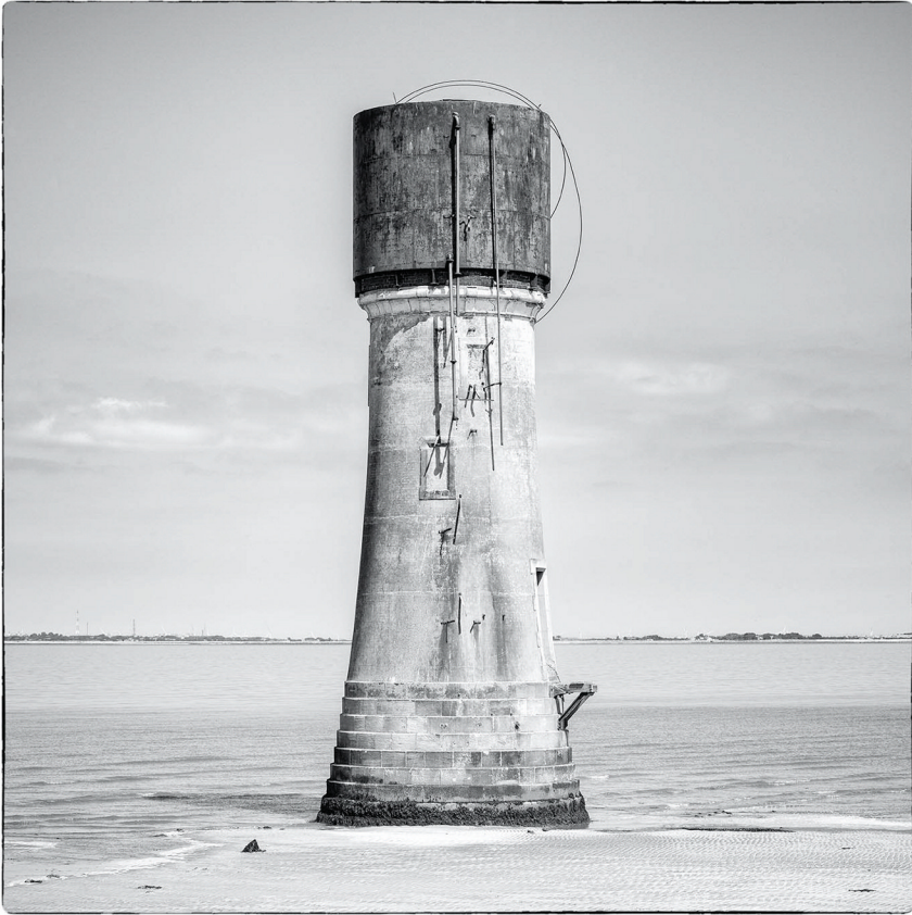
Spurn Point Water Tower
